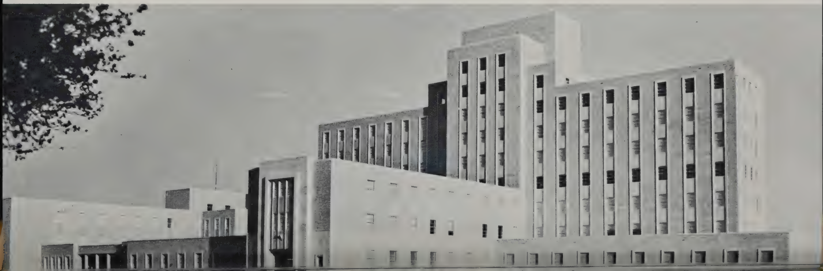
50. Methodist Memorial Hospital Before Construction of the 100-Bed Addition over the Foyer in the Foreground.
